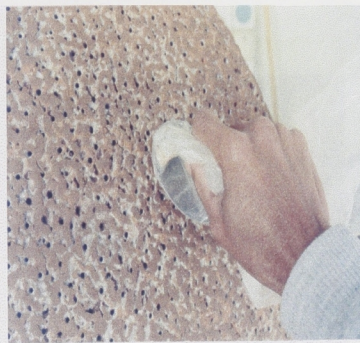
Fig.47 Using spoon wrapped with plastic for the second burnishing, this greatly brings out the shine on the surface.
