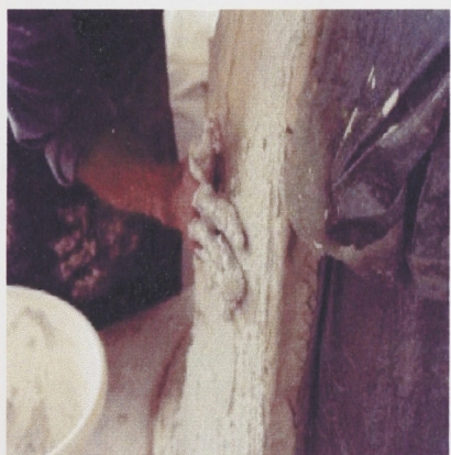
Fig.31 Applying the paper-plaster by hand on the dried slush coat.
