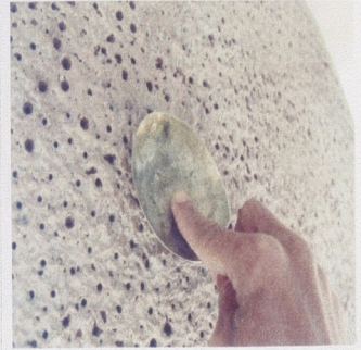
Fig.46 First burnishing is carried out by using the back of a spoon.
