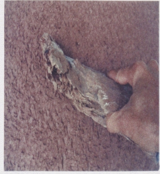
Fig.42 Texturing the entire surface with found objects such as tree branches and rocks.
